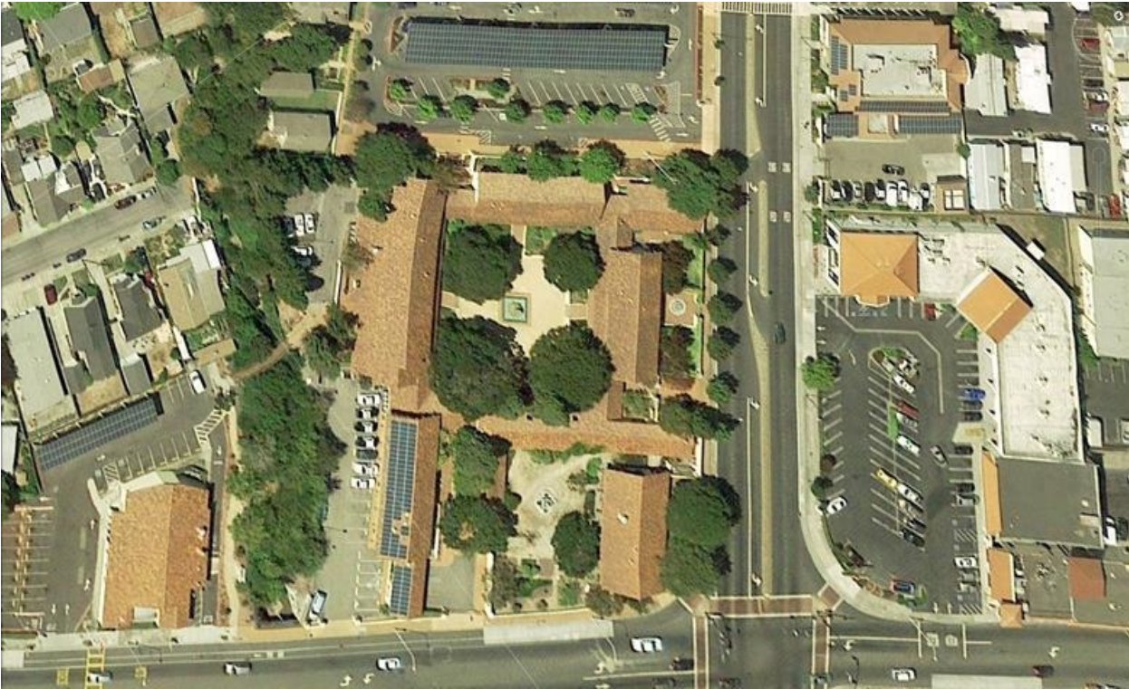
City Hall Building Roof Repair
