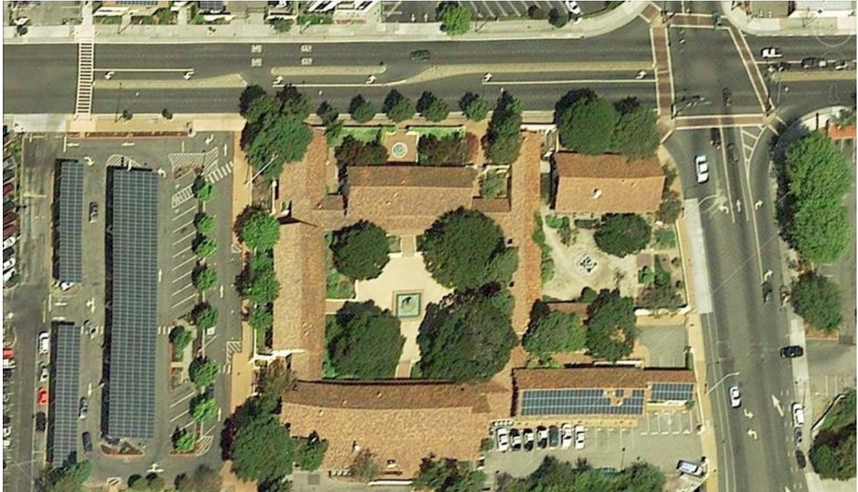
City Hall Main Courtyard paving and upper courtyard Pergola Project
